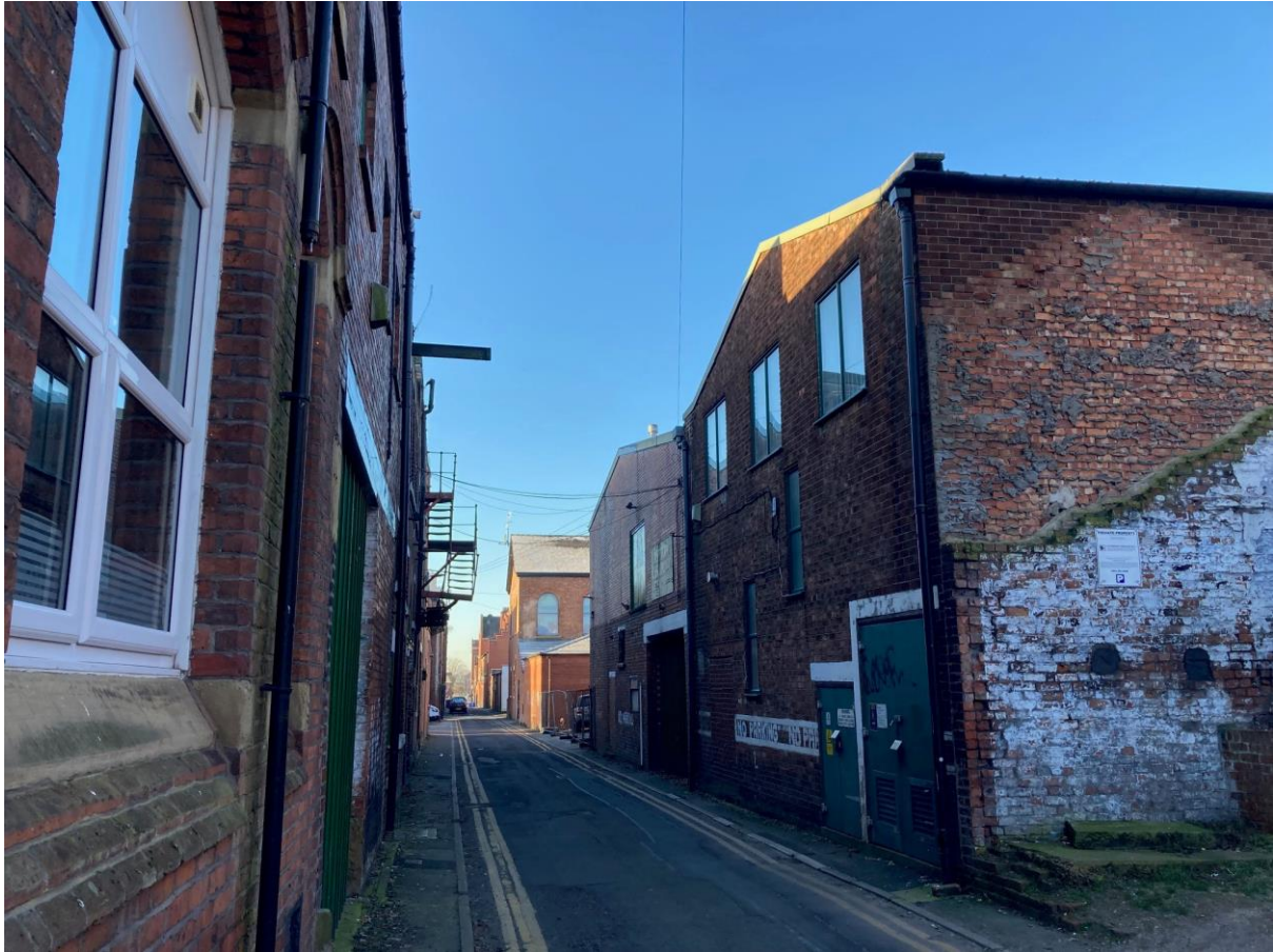
Photo 5: Rear of existing two storey outrigger, viewed from Fleet Street
