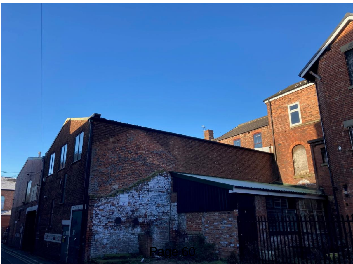
Photo 4: Existing building and two storey outrigger, viewed from Fleet Street
